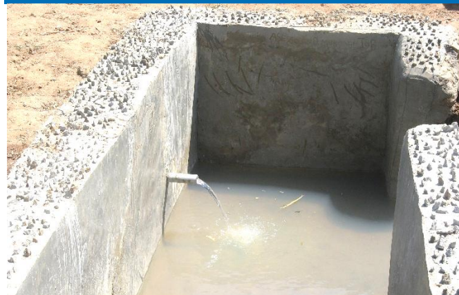
Spring after it was completed to be protected
